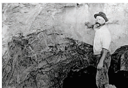
Wedderburn Old works North Royal George Mine. Original photograph caption: “Slide break on left. All mill ore, containing some dyke material, across the face. Looking south.”
